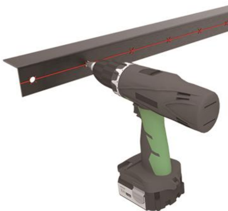
Pre-drill on the joist
