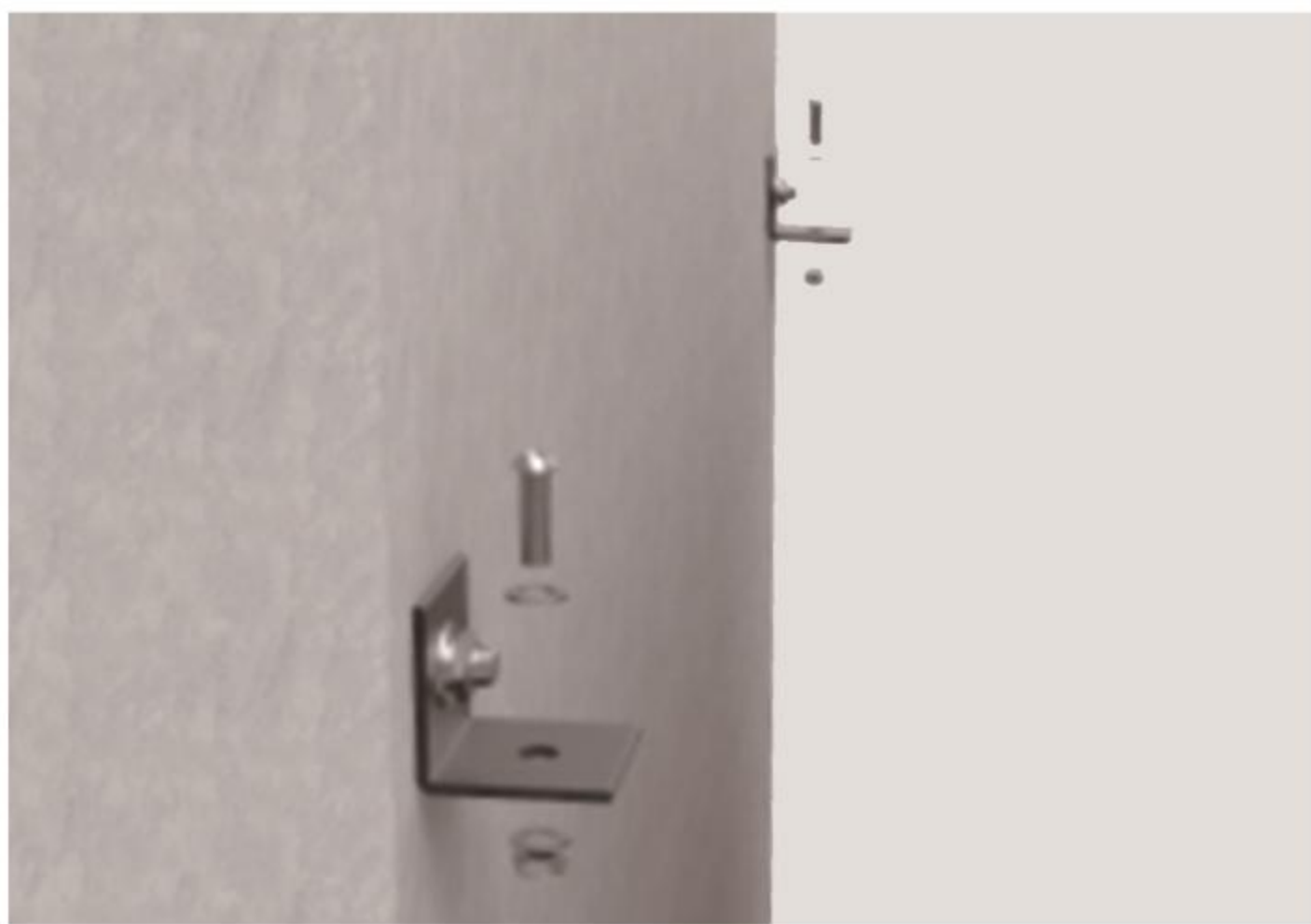
Fix the bracket to the wall
